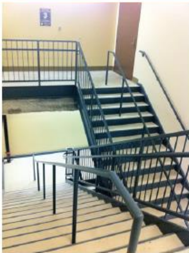
Enclosed exit stair with intermediate handrails.
